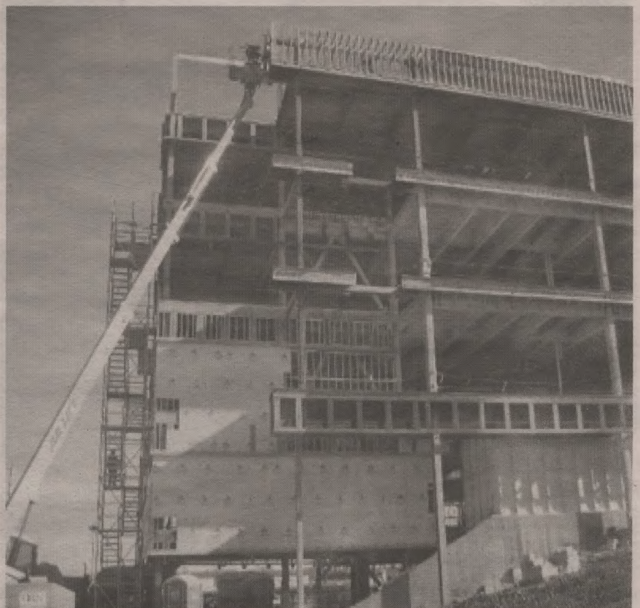
Construction the Center For Culinary Excellence.
